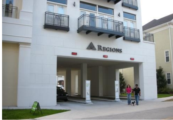
5 Figure 0-1: Drive-through integrated into a building
